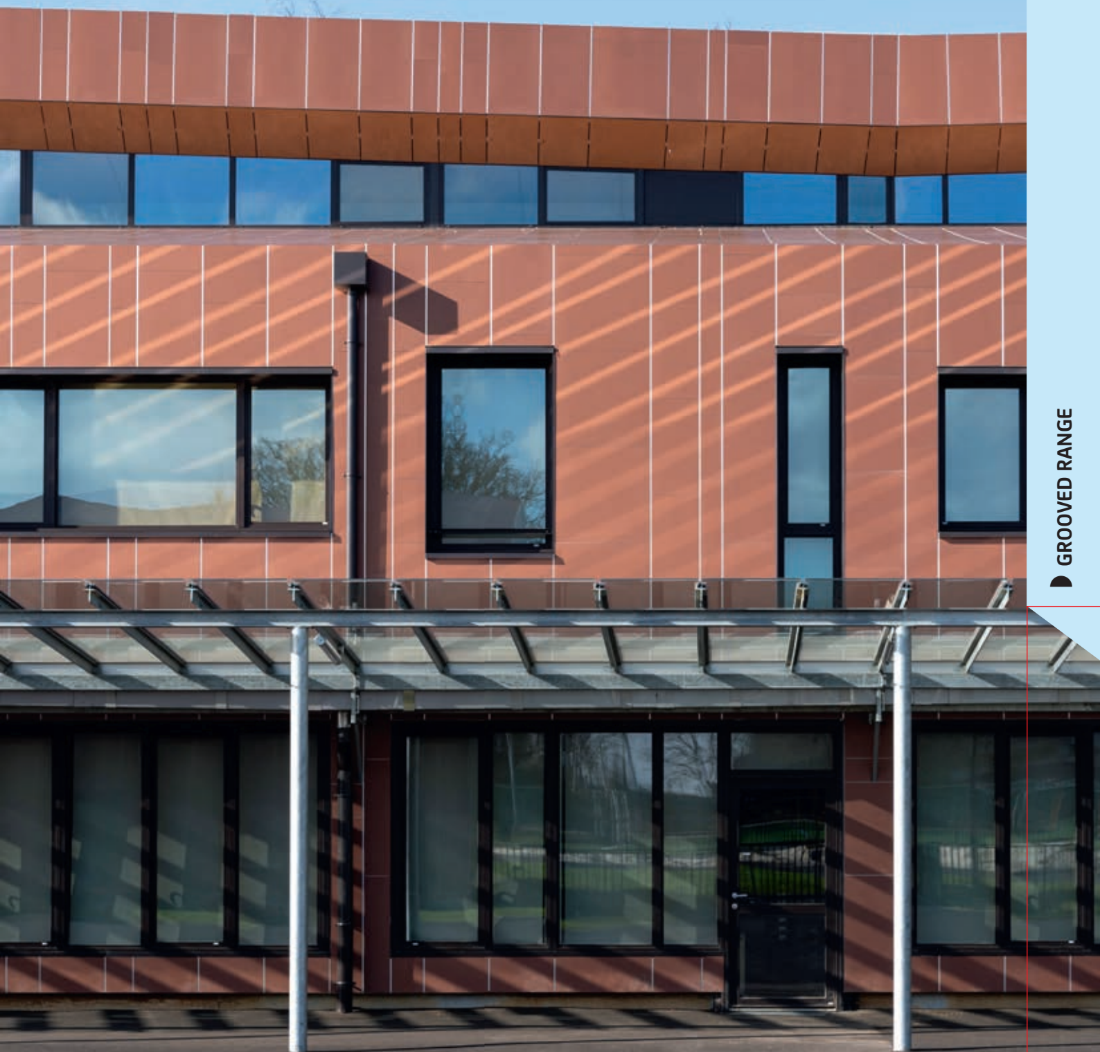
School Group Simone Veil, Evreux (FR) # Architects: Lebreton De Coquereaumont Architectes # Ardal & Acantha SMOOTH MATT, Copper (11-03) colour
