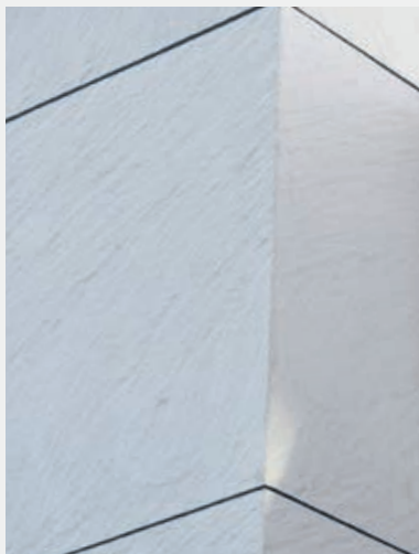
Single block bonded corner (BC)* *Made by the company on site
